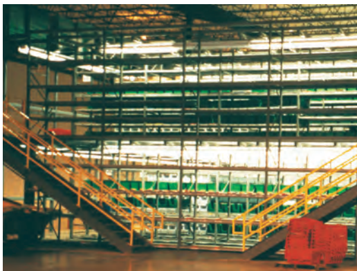
Multi-level Wide Span Pick Module
