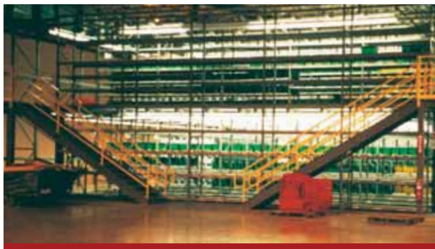
Multi-level Wide Span Pick Module
